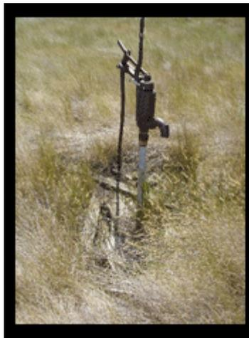
While the decommissioning procedure differs if the well in question is a small-diameter (drilled) well or a large-diameter (bored or hand-dug) well, it generally involves filling and sealing the well
