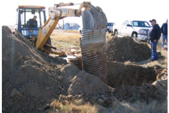
Figure 31: Removal of well casing
